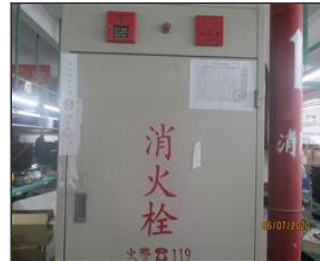
Photo of fire safety equipment 07 Fire alarm with fire hydrant.JPG
