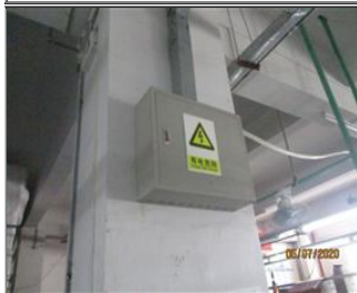
Photo of fire safety equipment 11 Electrical safety device with warning sign.JPG
