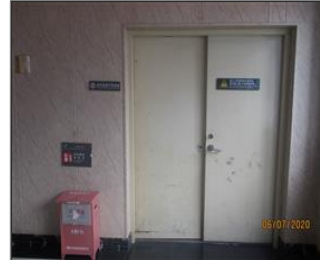
Photo of fire safety equipment 01 Fire door.JPG
