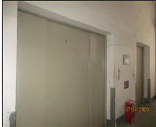
Photo of the inside of the main production hall 19 Cargo lifts.JPG
