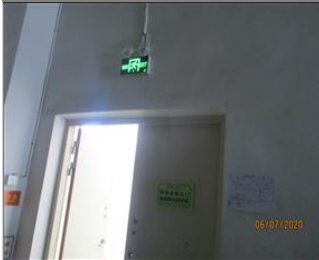
Photo of fire safety equipment 02 Exit door open outward.JPG
