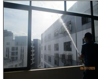
Photo of fire safety equipment 10 Testing fire hydrant.JPG
