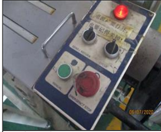
Photo of non-conformity NC 7.17 Control panels on the packing machines were only labelled in English language.JPG
