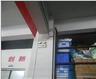
Photo of fire safety equipment 05 Emergency light for evacuation route.JPG
