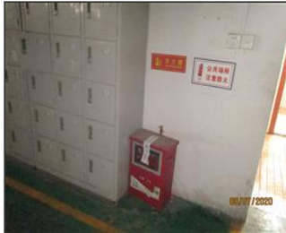
Photo of fire safety equipment 09 Fire extinguishers.JPG
