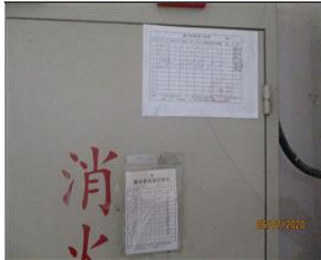
Photo of fire safety equipment 08 Inspection records of fire hydrant.JPG
