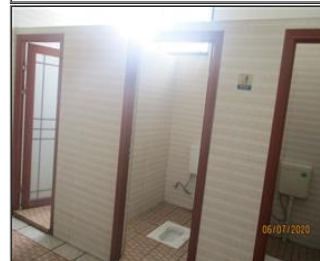
Photo of the sanitary facilities Toilet.JPG
