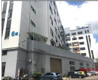
External photo(s) of the production unit(s) 01 Auditee on 6F of No.6 building.JPG
