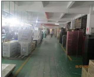
Photo of fire safety equipment 06 Evacuation route.JPG
