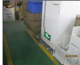
Photo of fire safety equipment 04 Exit sign for evacuation route.JPG
